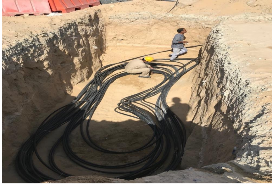
Figure 3.4: Trench of 2.5 m depth.
