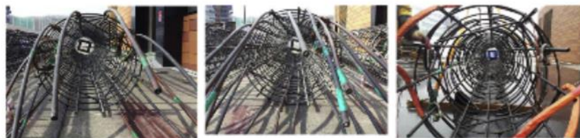
Figure 2.3: (a) 5-pair-parallel U-type (b) 10-pair-parallel U-type (c) S-type [55].
