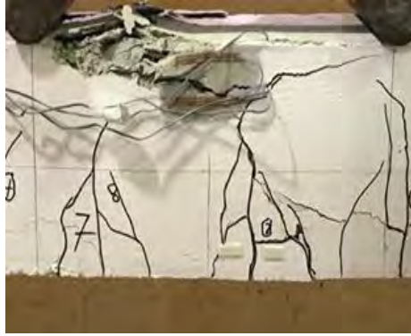
Figure 63: Failure mode of beam 2B8EC.
