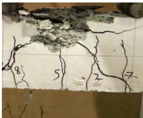
Figure 66: Failure mode of beam 2B12EC.
