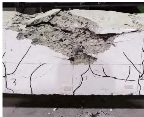
Figure 58: Failure mode of beam 2G20ER.
