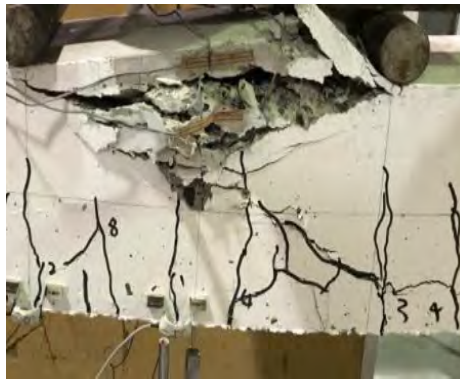
Figure 68: Failure mode of beam 3B16EC.
