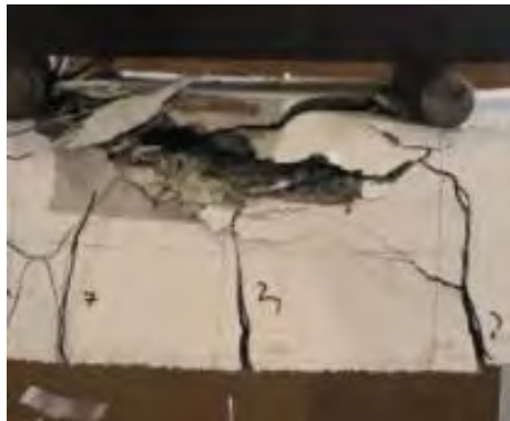
Figure 64: Failure mode of beam 2B10EC.
