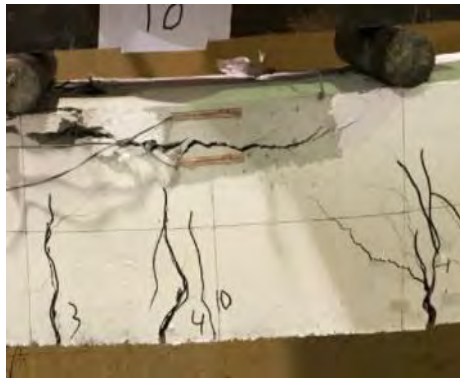
Figure 60: Failure mode of beam 2G10UR.
