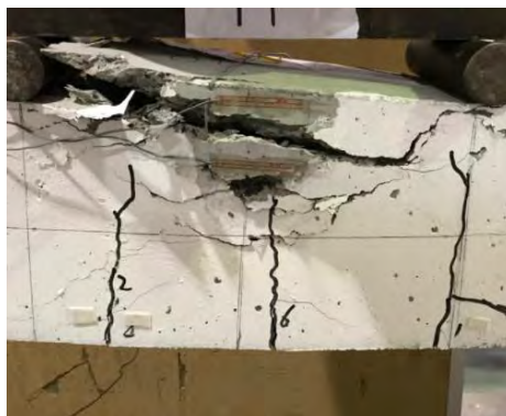
Figure 69: Failure mode of beam 2B20EC.
