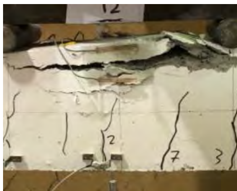
Figure 62: Failure mode of beam 2G26UR.
