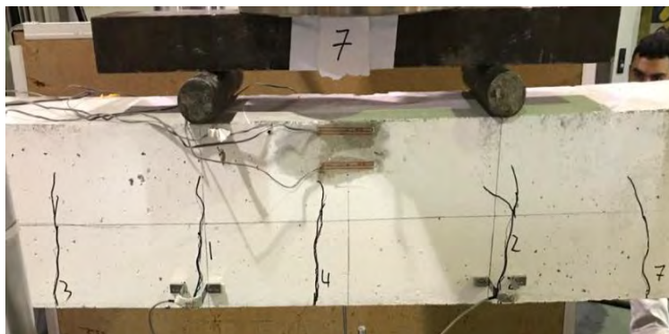
Figure 80: Cracks propagation of beam 2G10ER.
