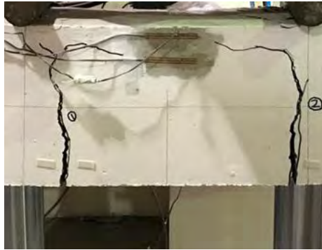
Figure 51: Failure mode of beam 2G8EC.
