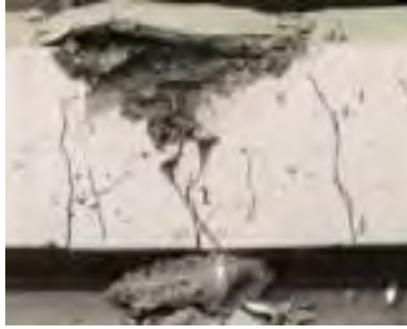
Figure 67: Failure mode of beam 2B16EC.
