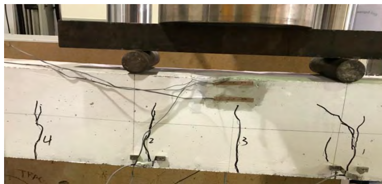
Figure 75: Cracks propagation of beam 2G10EC.
