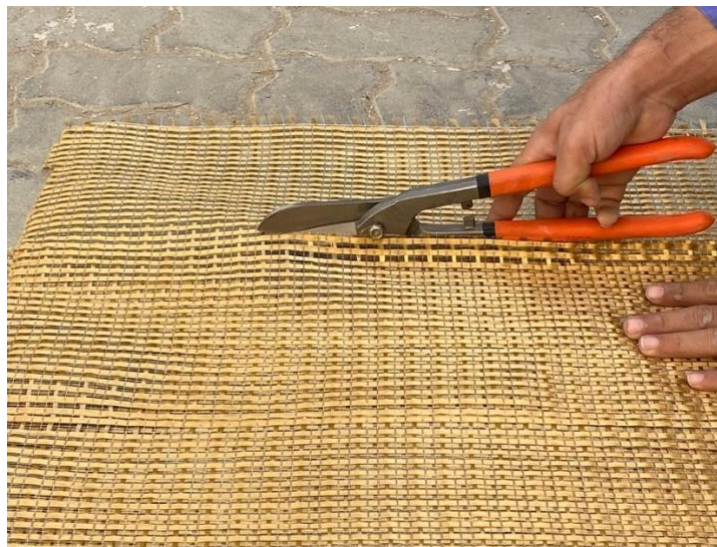
Figure 22: Mesh preparation process.
