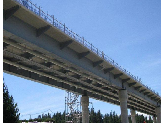
(b) Steel girders
