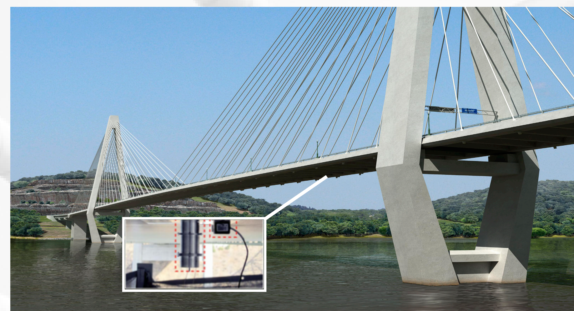
Figure 2: Photograph of the PFIG mounted next to a Crossbow accelerometer underneath the bridge girder photo (3)
