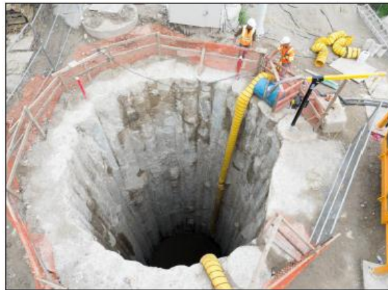
Figure 2. Circular secant pile wall – Compression Ring
