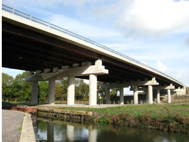
Figure 7: Example of composite steel girder bridge [7]
