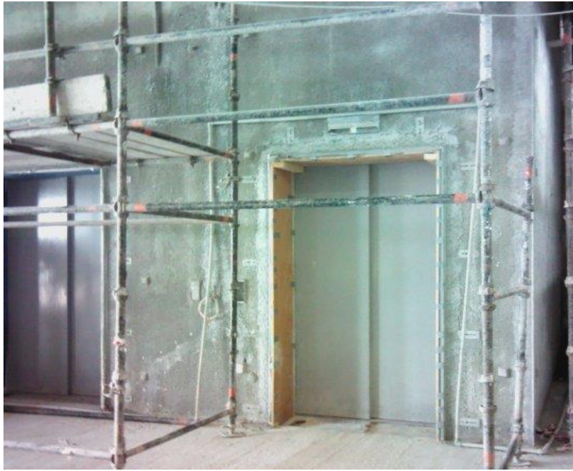
Figure 19: Digital image of concrete wall with door and some steel scaffolding
