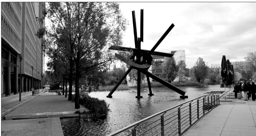
Fig. 4 Rainwater treatment system in Potsdamer Platz, Berlin
