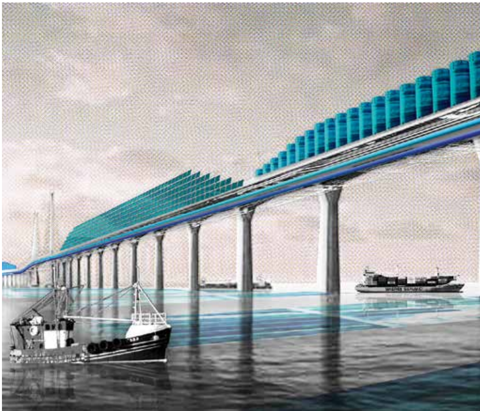
Figure 9. A rendering of the HZMB with linear arrays of solar panels and water storage tanks.
