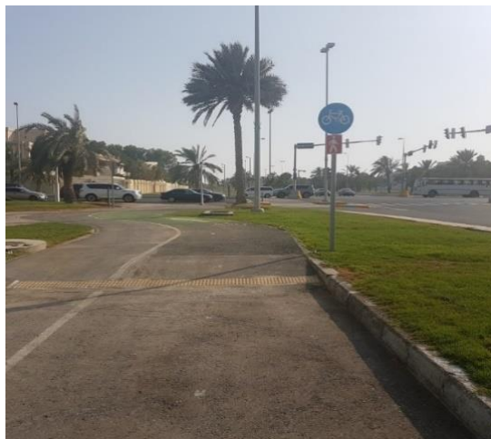
Figure 34 bicycle Lane, Al Khaleej Al Arabi street, U.A.E.
