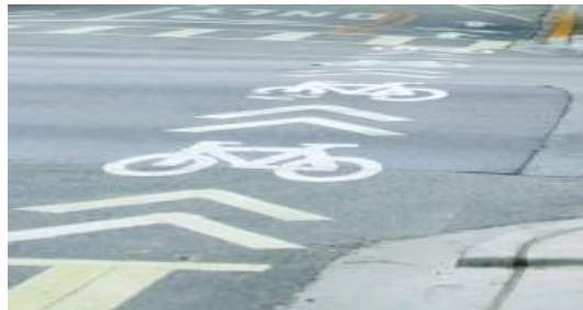
Figure 36 Intersection crossing marking [90].
