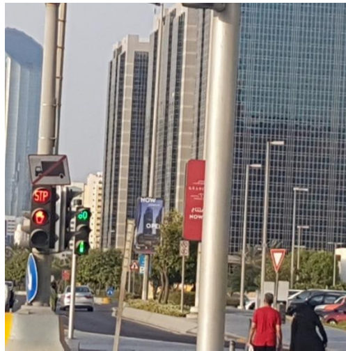
Figure 30 Pedestrian traffic signal with countdown timer, Al Corniche street, U.A.E.
