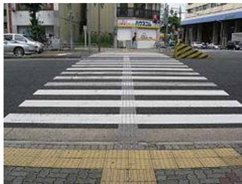
Figure 32 Directional warning tactile ground surface indicators [87].
