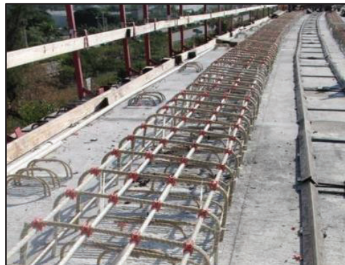
Figure 2: Miami-dade metrorail project used GFRP bar reinforcement [10]
