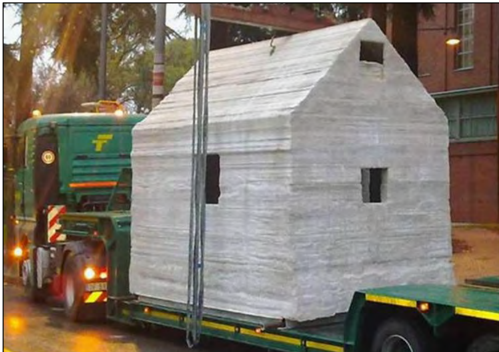
Figure 13: Single Room Printed using D-shape technique [29].
