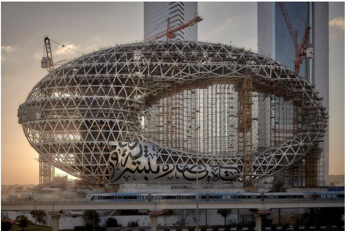
Figure 6-2: Dubai Future Museum under Construction [57]
