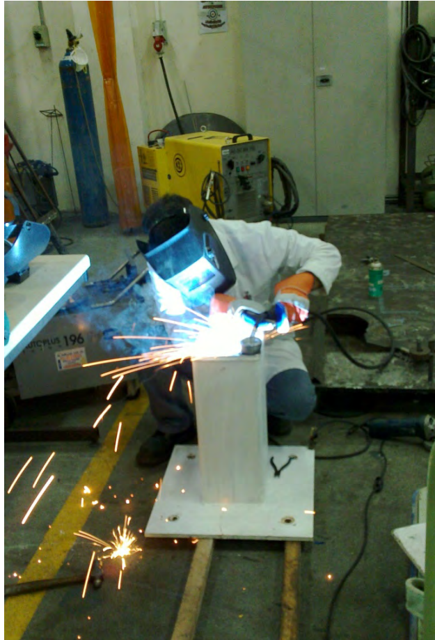
Welding of sphere holder on column head
