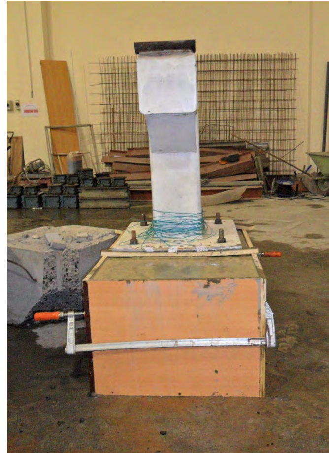
Concrete poured in the formwork
