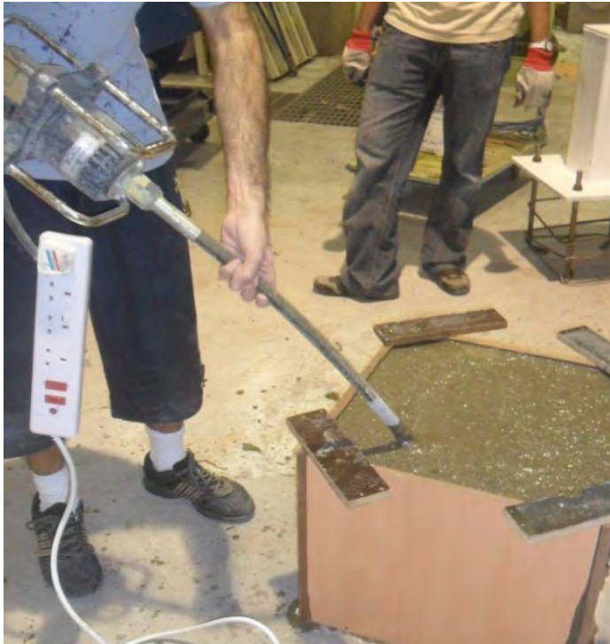
Vibration of Concrete
