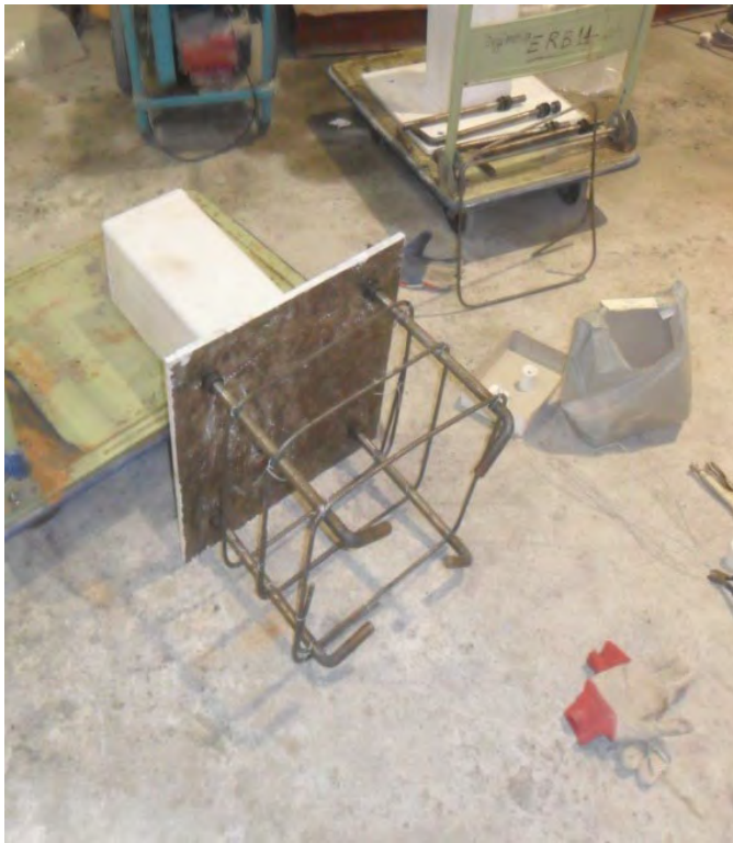
Tying of Stirrups/ties
