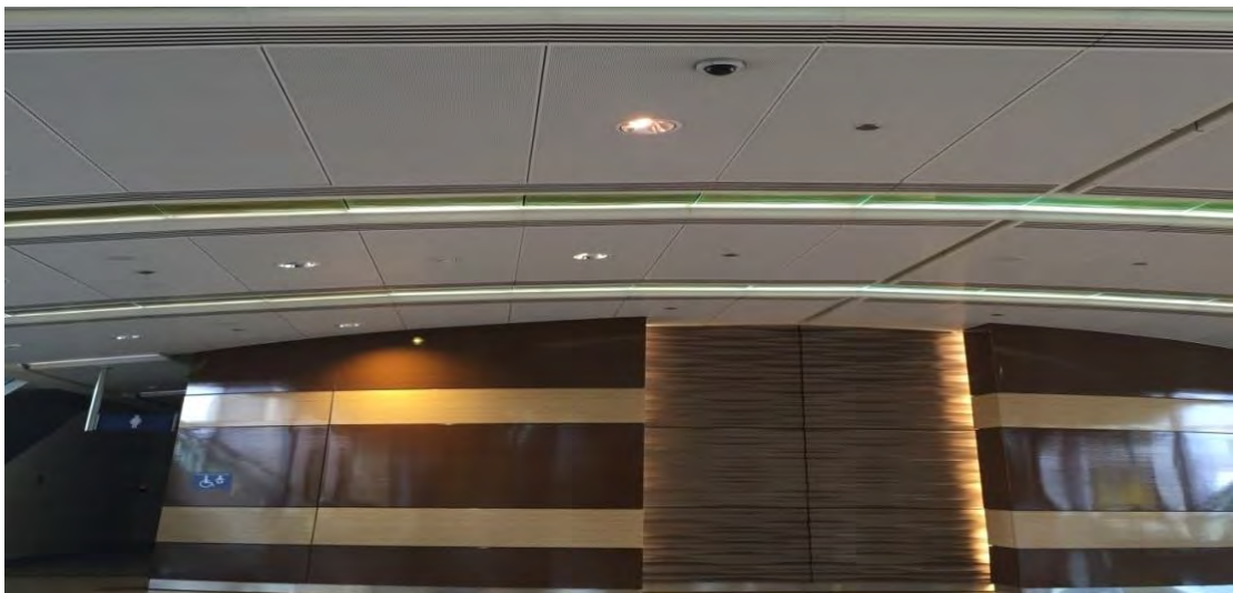
Figure 12: LED Lighting System in Dubai Metro Stations
