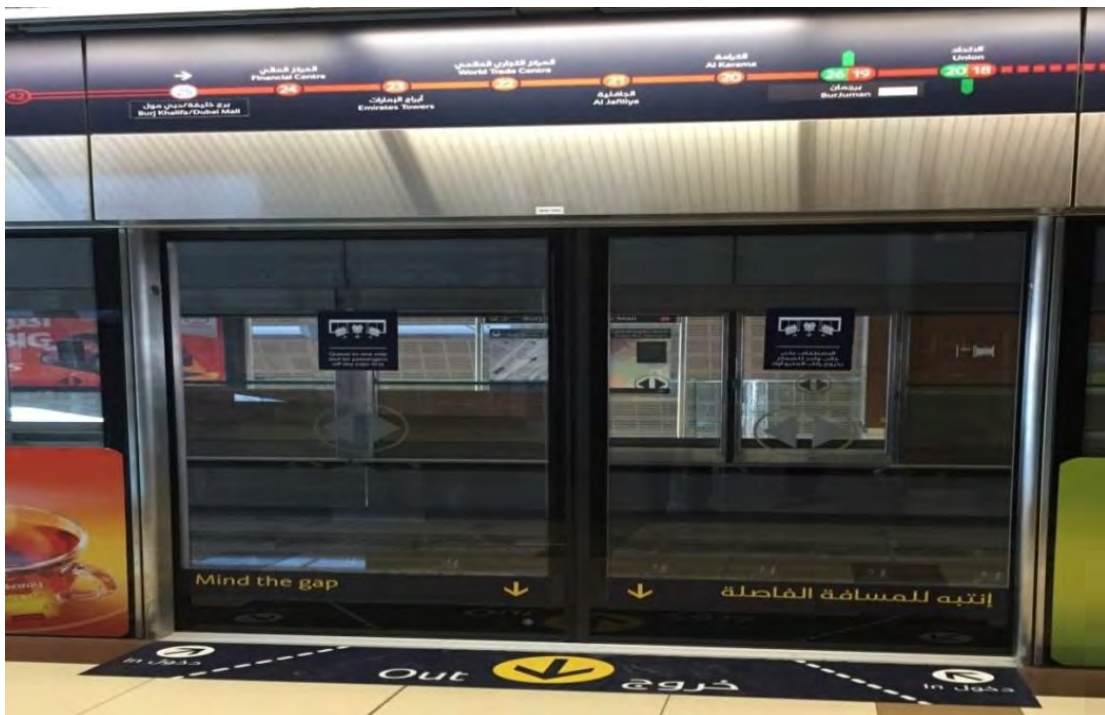
Figure 9: Fully Closed PSD in Dubai Metro Stations
