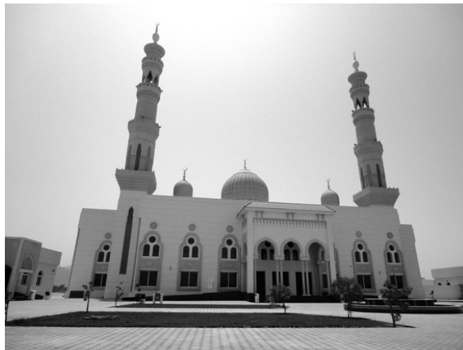
Figure 1. Photo of the mosque used for the study
