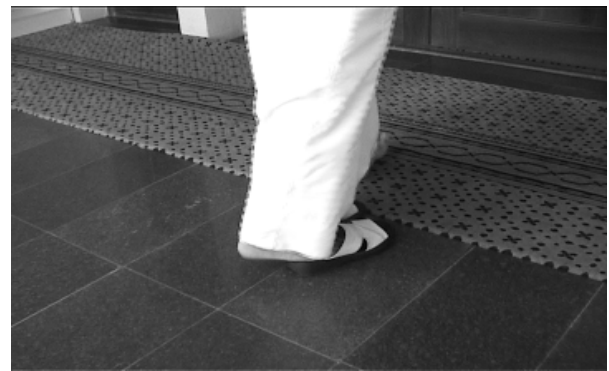
Figure 5: The change of material visually defines the separation between clean and non-clean zones.
